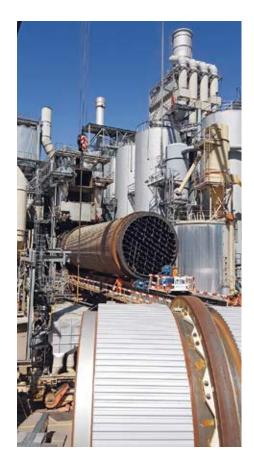
The old drum is moved out, the new drum is ready to be installed
