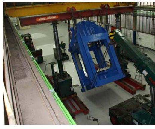
Insertion of the one-piece press body consisting of nodular graphite cast iron
