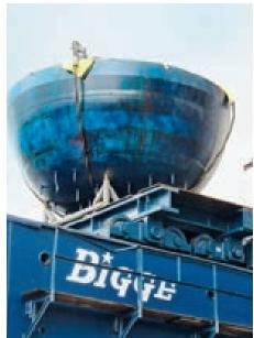
Transport of the reactor floor (calotte)
