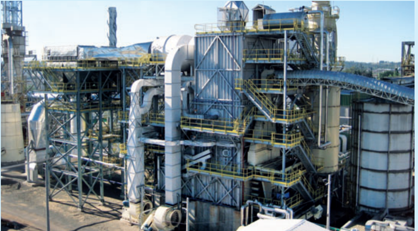
SES energy plant in Chile
