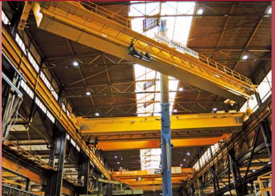
The crane is put into position
