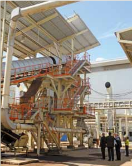
Tour of the outside facilities
