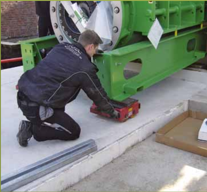
Generator during installation inside the building
