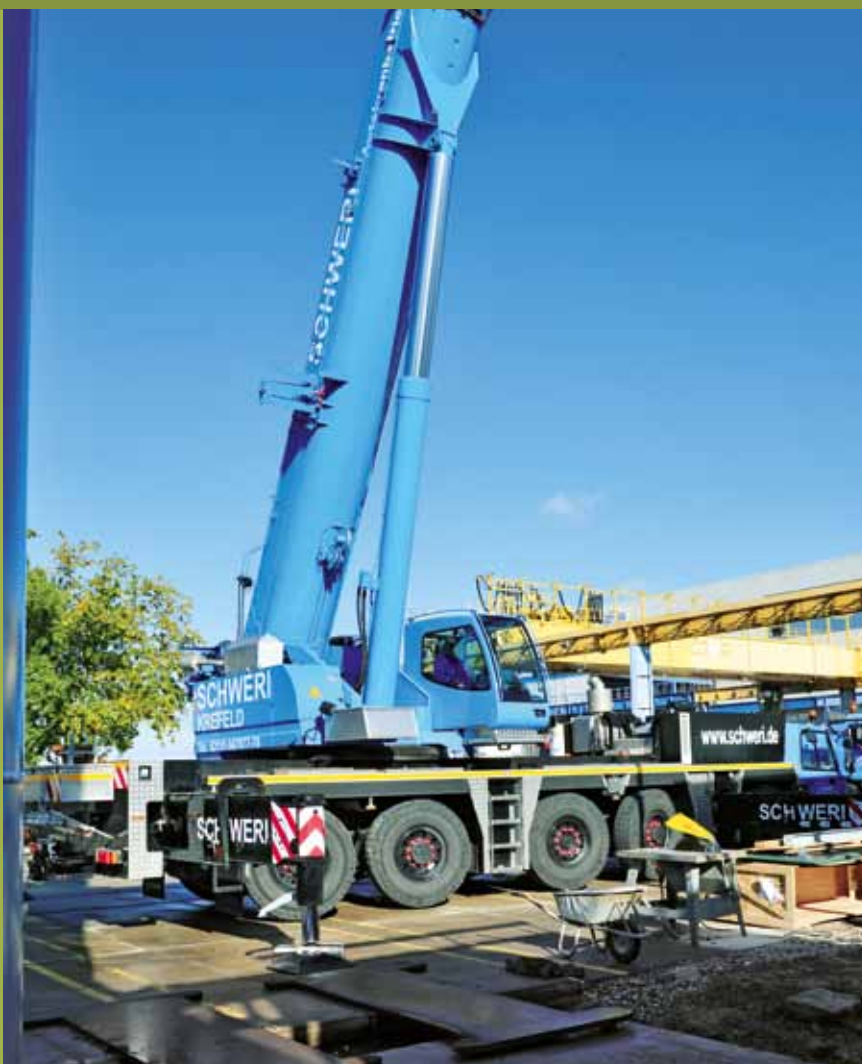
Work at the location
