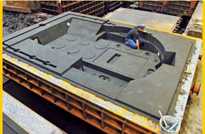
Molding works for the prototypes
