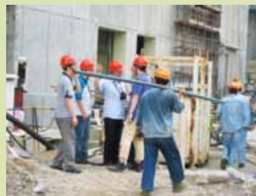
NPP construction site in China
