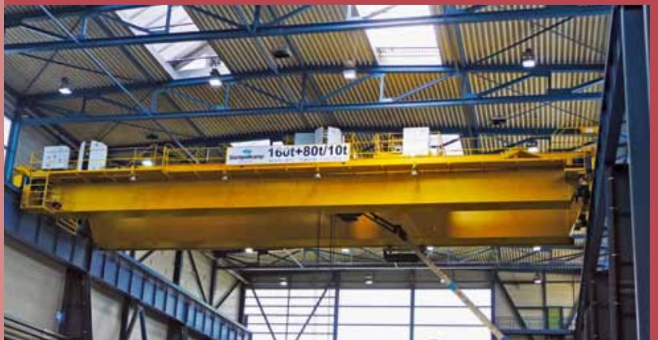
Up in the air – finished!
