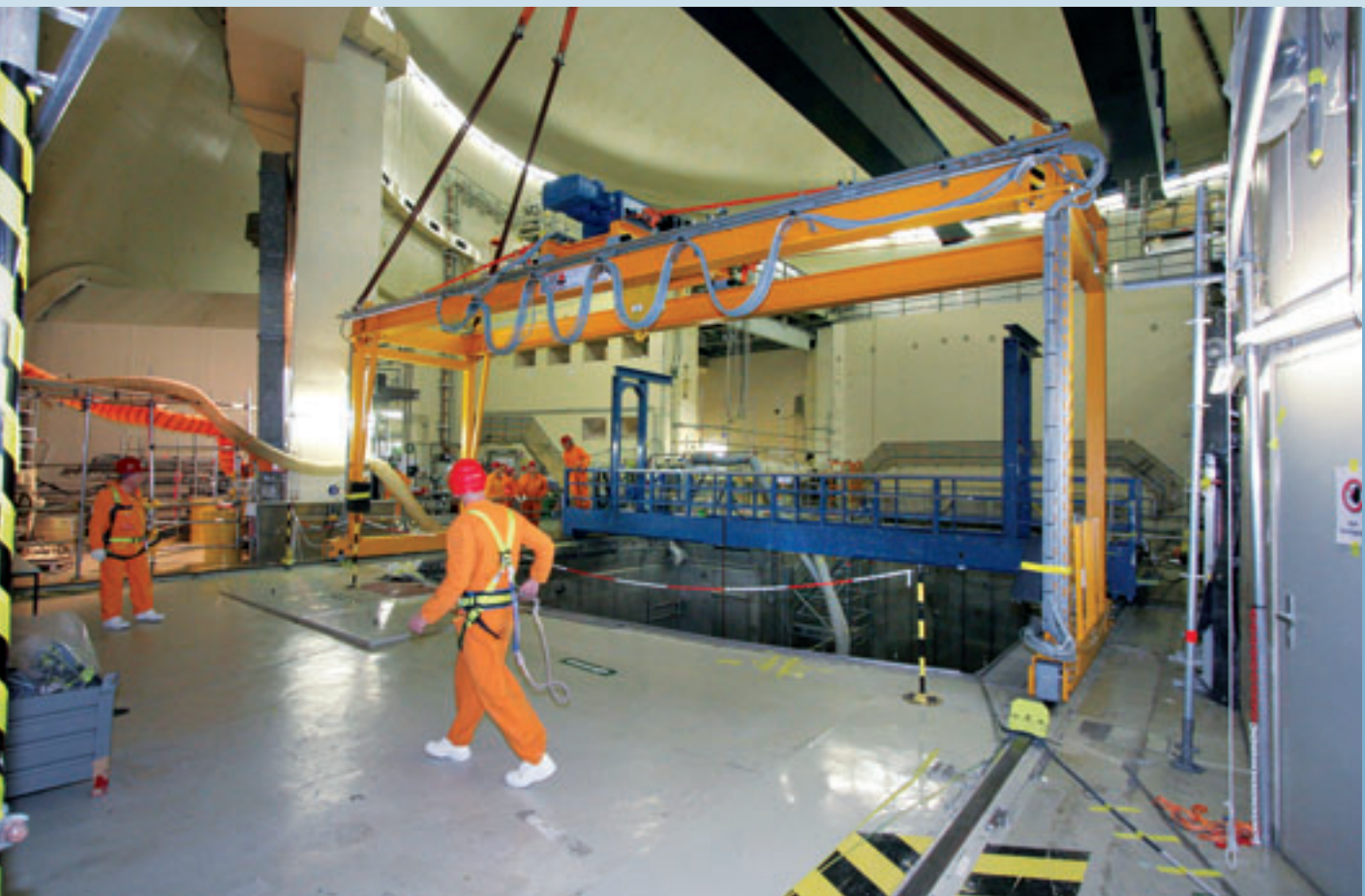
The crane on four pillars inside the control zone
