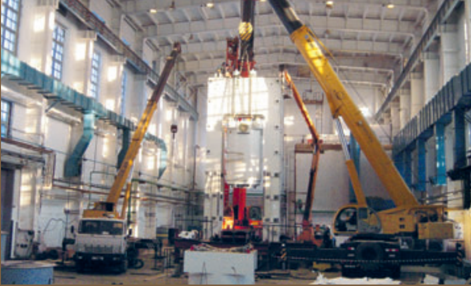
Installation of the upper cylinder
