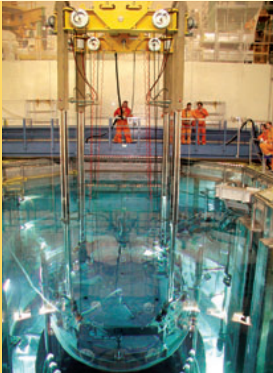
Transport of the RPV sealing head with the multi-purpose lifting device
