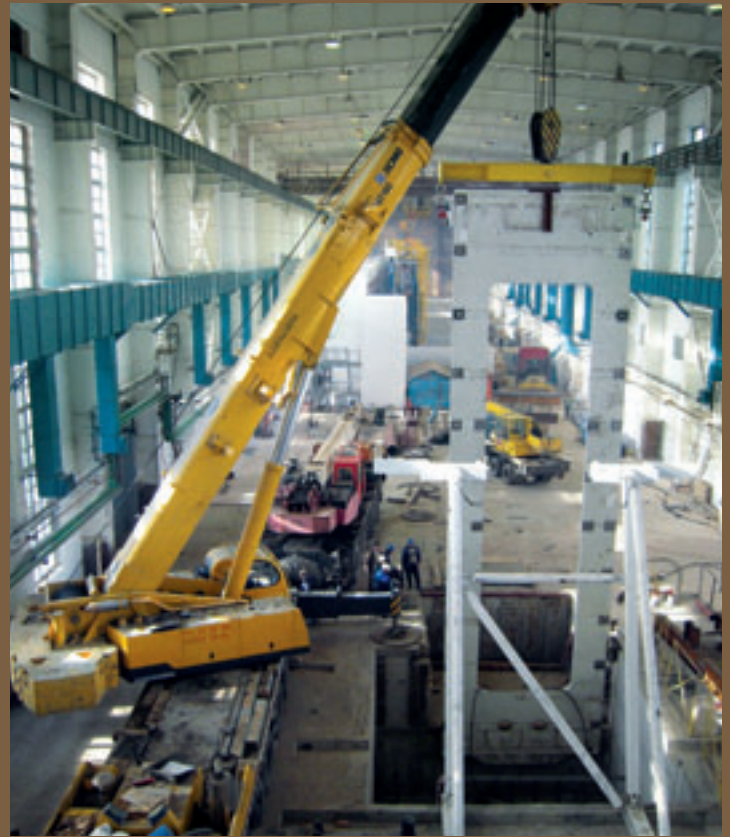
Installation of first frames
