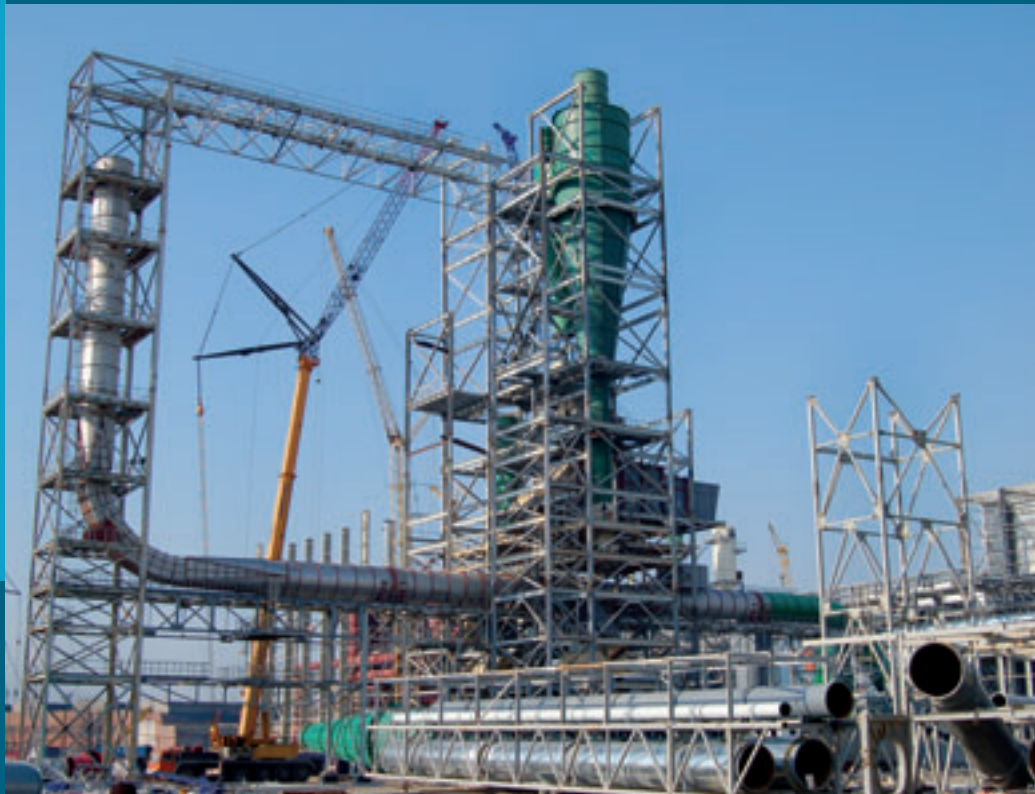
Installation of the fiber dryer
