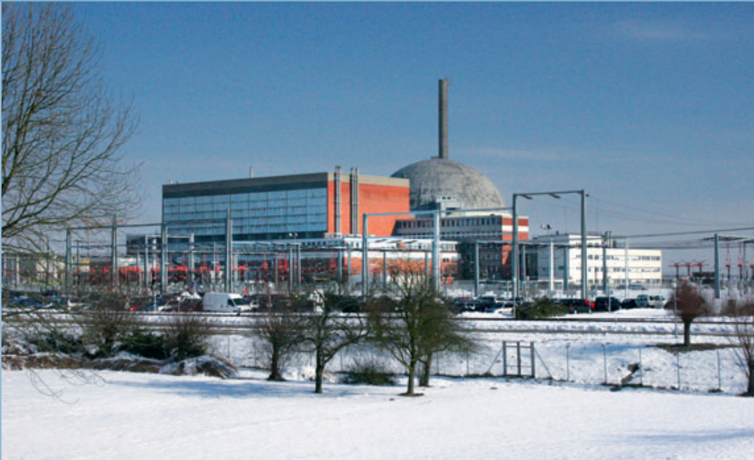
The nuclear power plant Stade during the dismantling procedure
