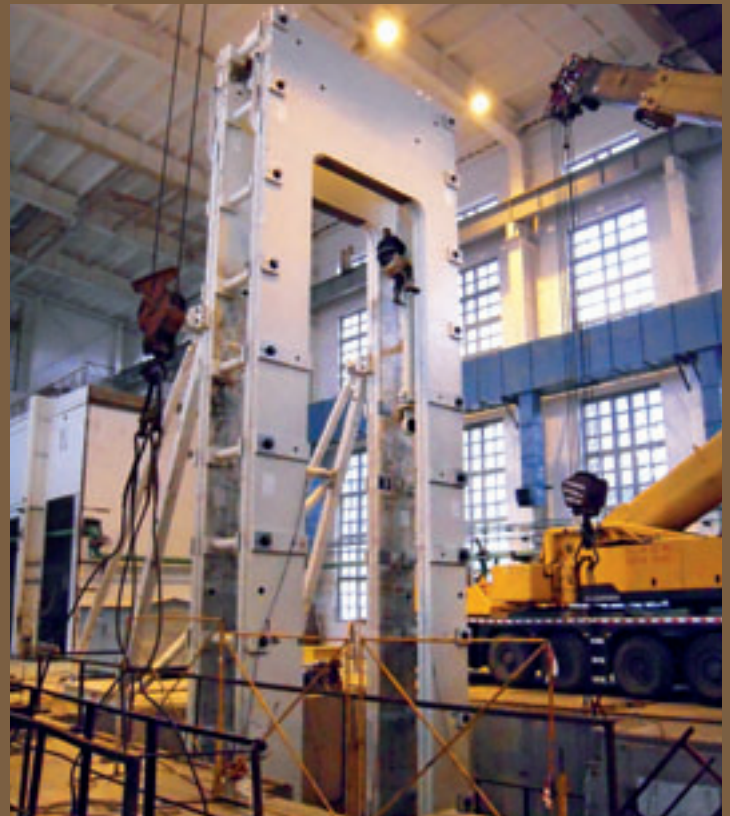
The press frames are installed
