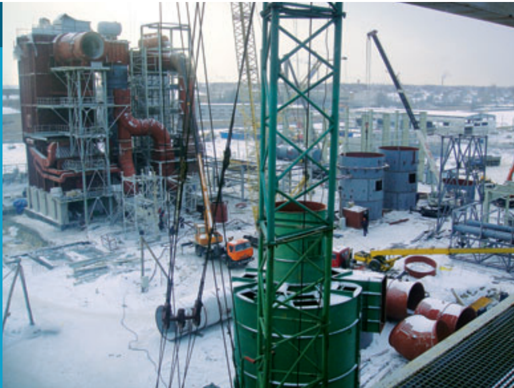
Snow and coldness at the construction site
