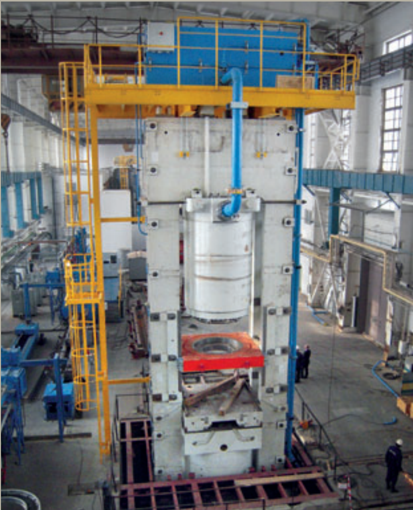
The shell construction of the press is finished
