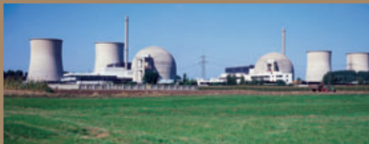
Installation of hydrogen recombiners at the nuclear power plant Biblis
