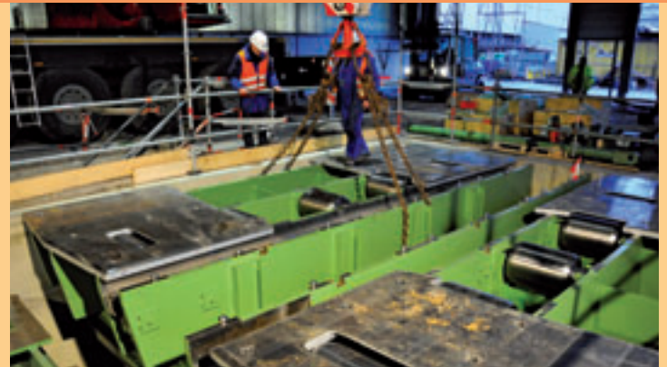
Installation of roller tables
