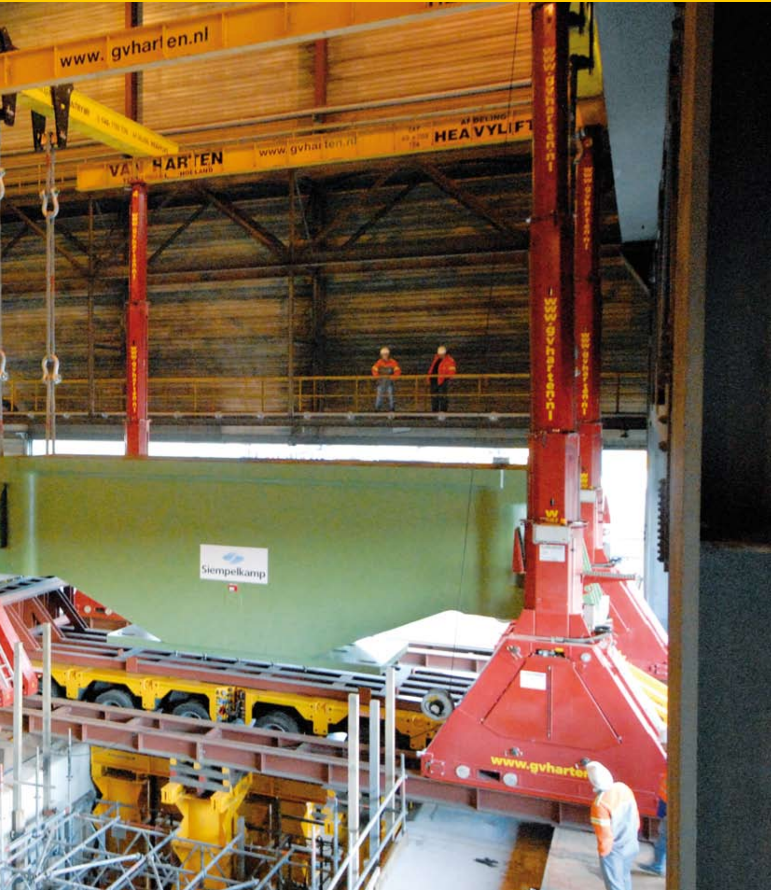
Lower bolster for the press at the building site
