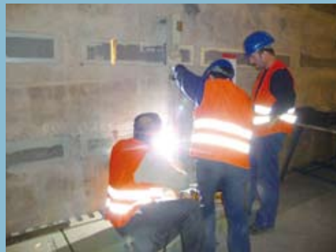
Welding on of supports for the wall elements
