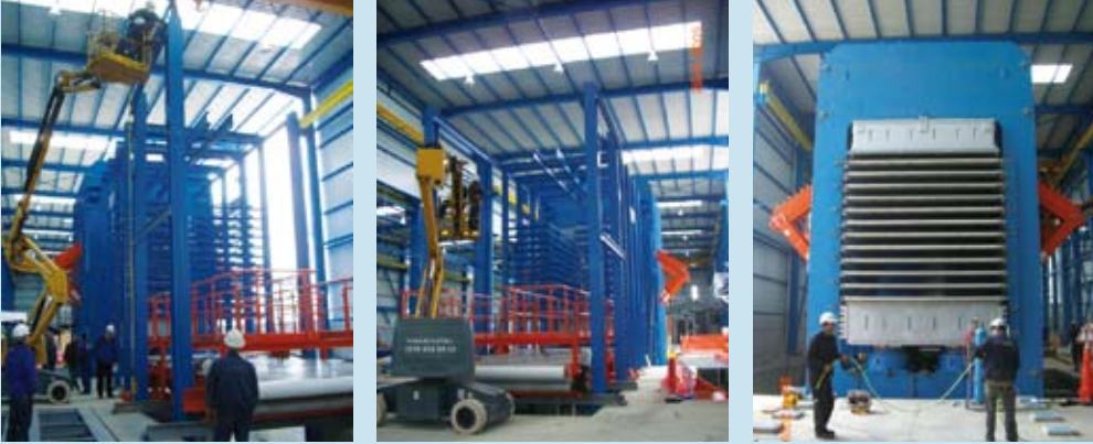
Assembly of press and loader and unloader unit
