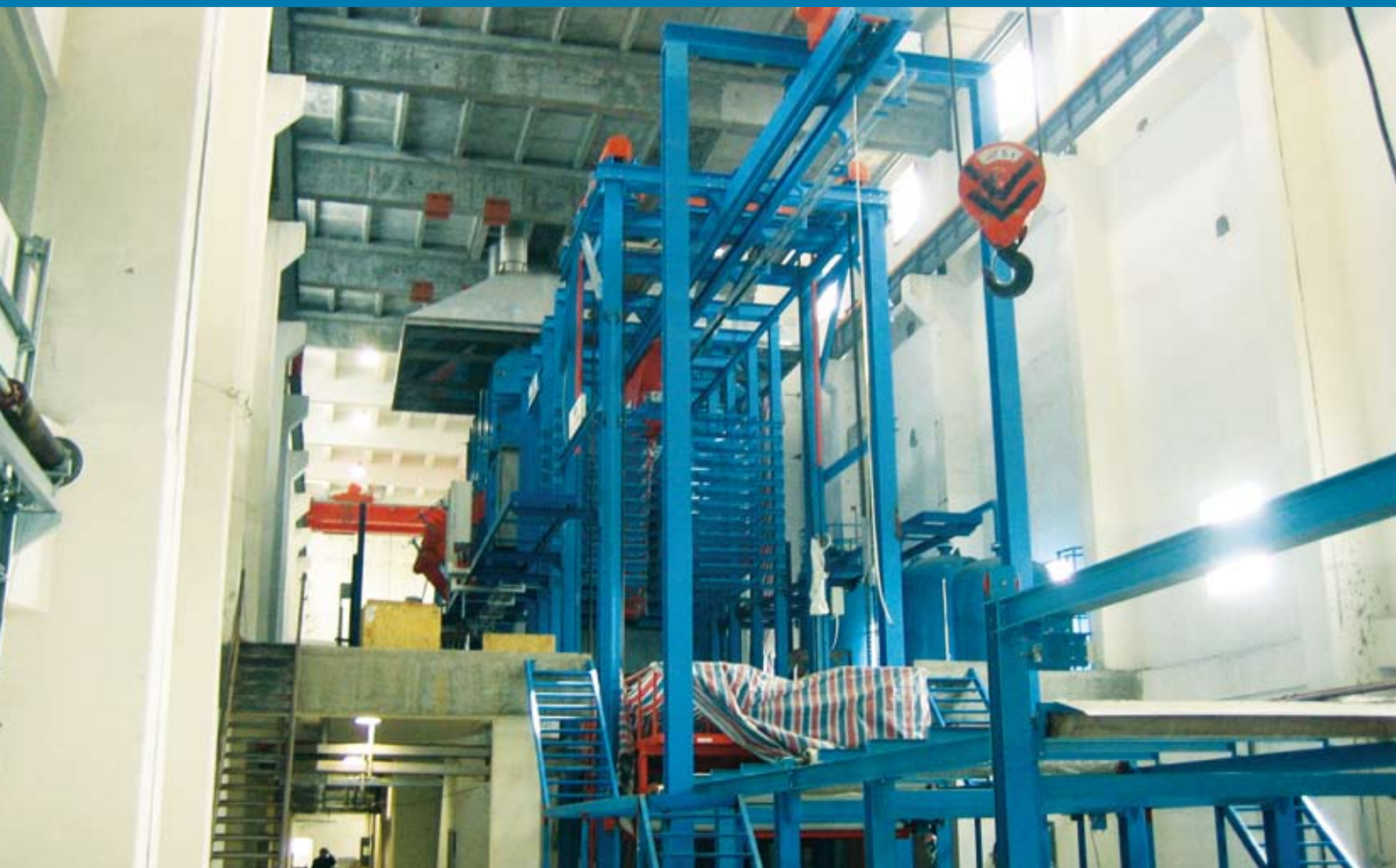
Complete plant during assembly
