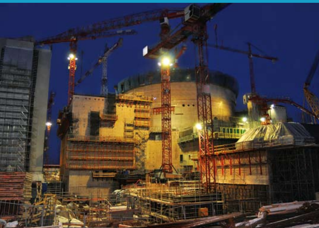
Construction site of EPR reactor in Finland
