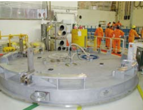
Pressure vessel head consisting of two segments and centering cantilevers
