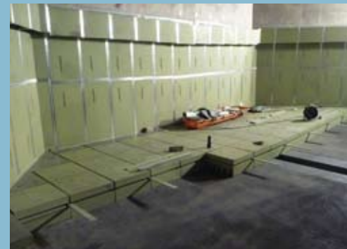
Installation of the 578 Core Catcher floor elements
