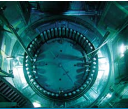
The sealing lid seals the open reactor inside the flooded pond
